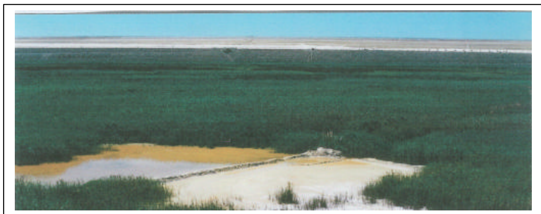
Figure 8(b): Leachate from the slimes dam above with the other slimes dam in the background
